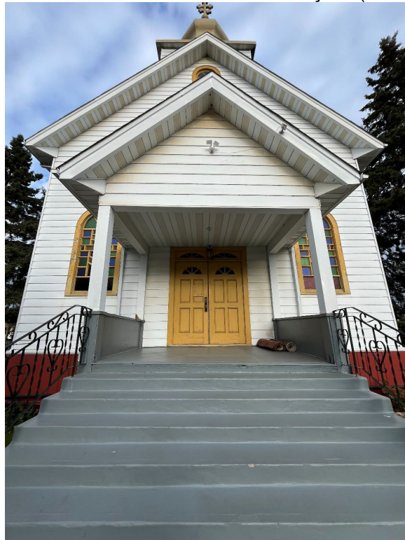
Photograph 8: West elevation entrance to the church (Source: Egis, October 15, 2025).
