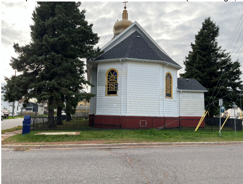
Photograph 4: East elevation of 716 Pacific Avenue showing the apse end facing McPherson Street between Pacific Avenue and Connolly Street (Source: Egis, October 15, 2025).
