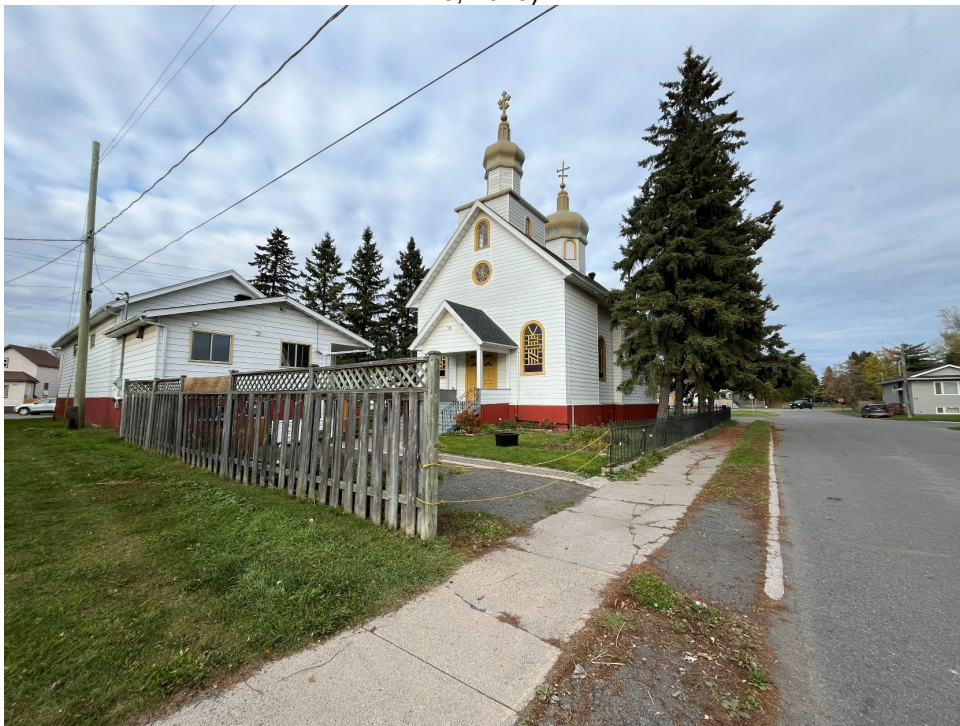
Photograph 2: Southwest corner of 716 Pacific Avenue from Connolly Street (Source: Egis, October 15, 2025).
