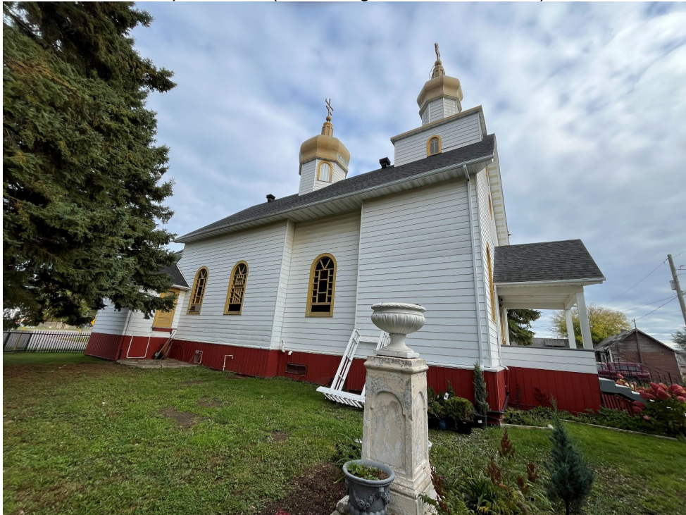
Photograph 6: View of the north elevation of 716 Pacific Avenue showing concrete monument in the garden (Source: Egis, October 15, 2025).
