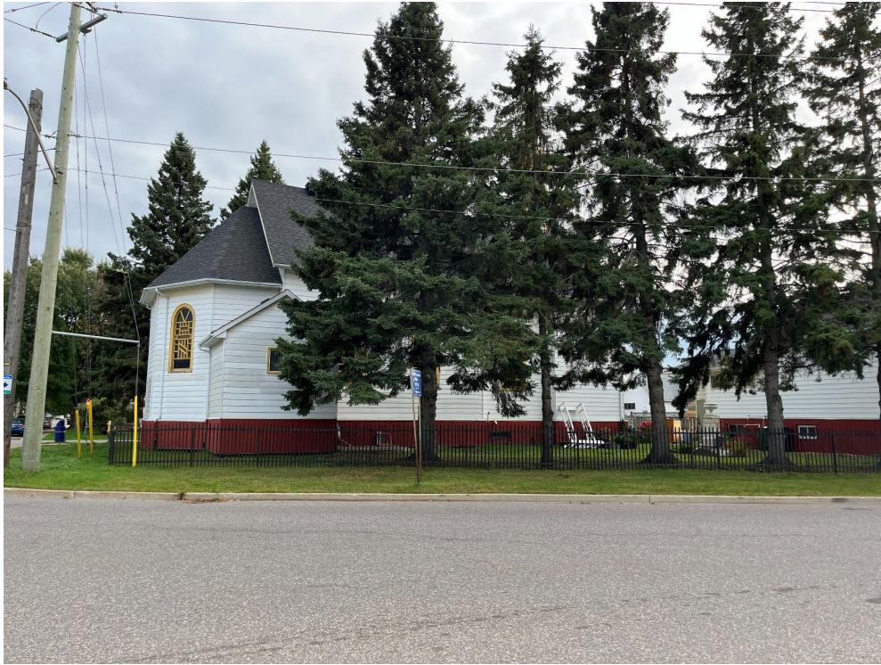
Photograph 5: View from Connolly Street of the south elevation of 716 Pacific Avenue screened by row of spruce trees (Source: Egis, October 15, 2025).
