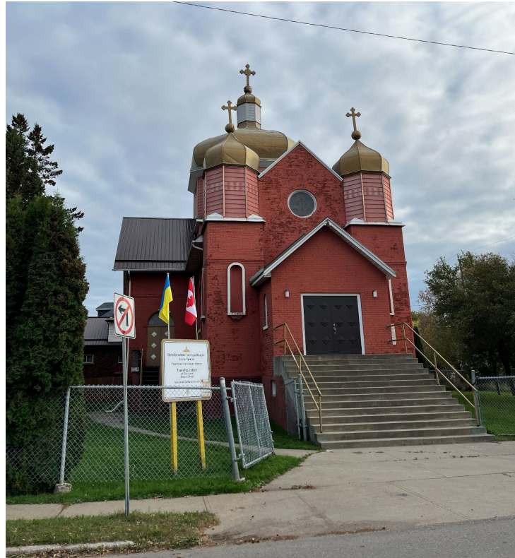
Photograph 13: View of the Ukrainian Catholic Church of Transfiguration at 629 McIntosh Street (Source: Egis, October 15, 2025).
