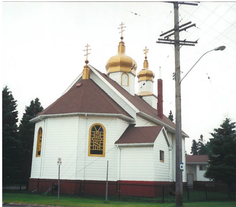
Image 4: Colour photograph of the church after renovations (Source: City of Thunder Bay)
