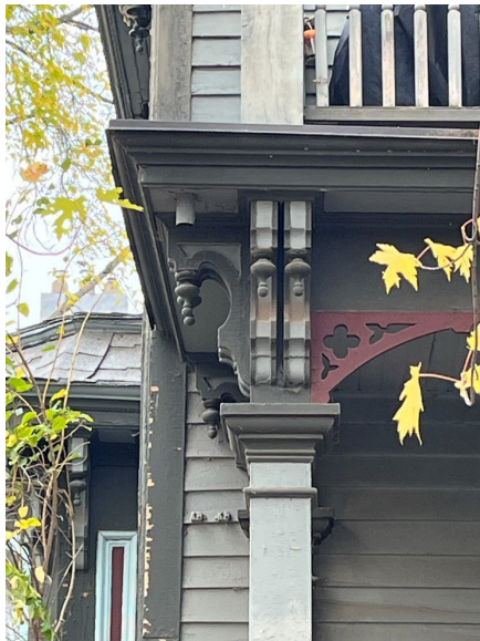
Photograph 13: Decorative details of the porch (Source: Egis, October 15, 2025).
