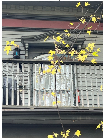
Photograph 14: Close-up of second-storey balcony balustrade (Source: Egis, October 15, 2025).
