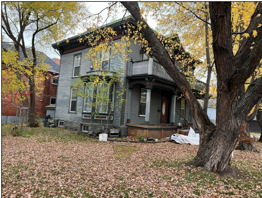
Photograph 7: West and south elevations from the sidewalk (Source: Egis, October 15, 2025).
