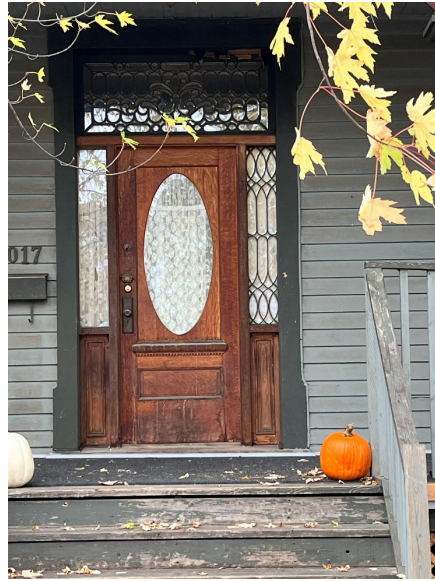
Photograph 16: Close-up of the front entrance featuring original wood front door with square-headed transom and sidelights (Source: Egis, October 15, 2025).
