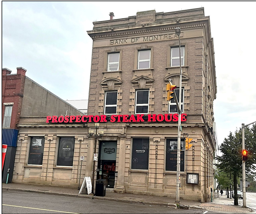
Photograph 2: West elevation (former bank entrance) of the building (Source: Egis, October 17, 2025).
