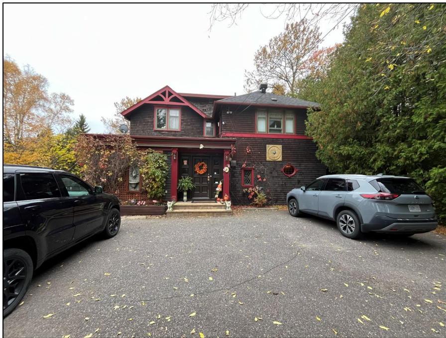
Photograph 1: North elevation (current front façade) of the house (Egis, October 16, 2025).
