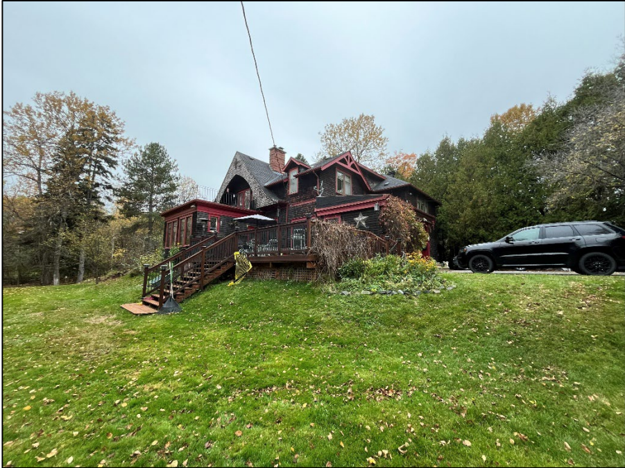
Photograph 3: North and east elevation of the house (Egis, October 16, 2025).
