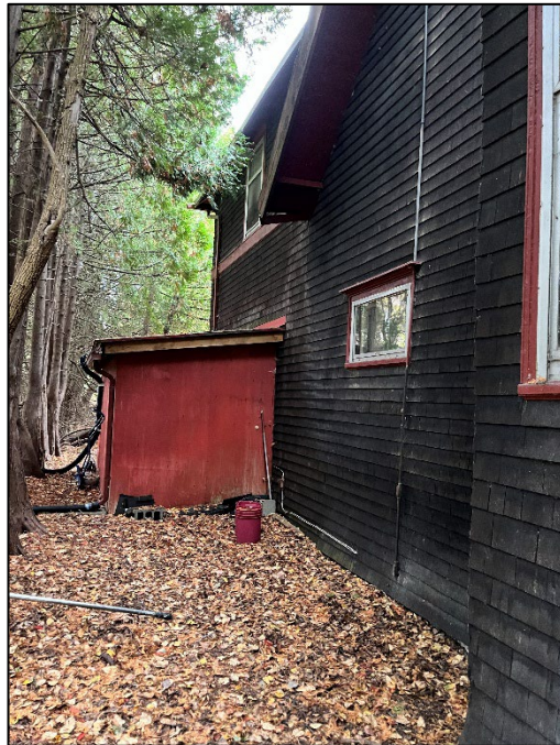
Photograph 8: West elevation, looking north (Egis, October 16, 2025).
