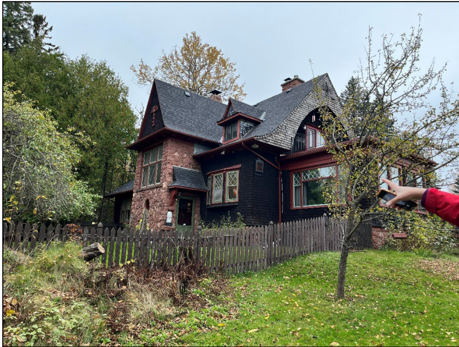
Photograph 6: South and east elevation of the house (Egis, October 16, 2025).
