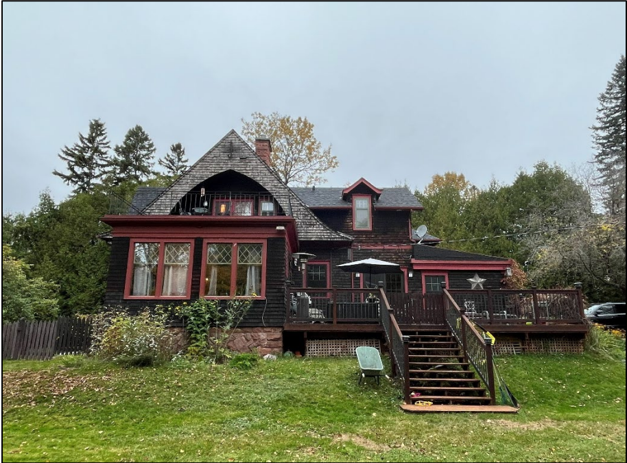
Photograph 2: East elevation of the house (Egis, October 16, 2025).
