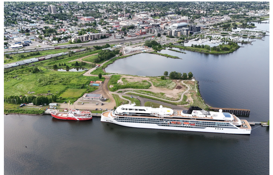
Figure 16. Improvements to the cruise ship wharf
