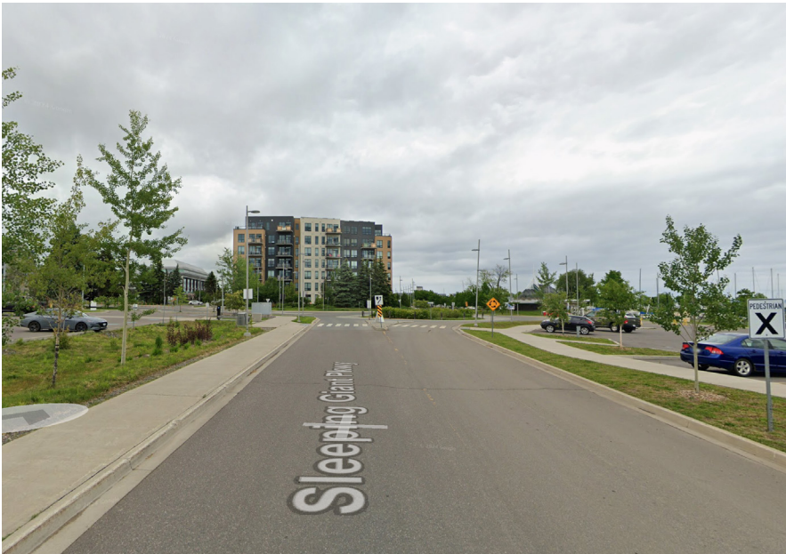
Figure 13. Construction of the first southerly leg of the Sleeping Giant Parkway
