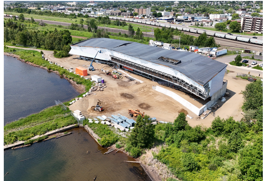
Figure 14. The Thunder Bay Art Gallery (currently under construction)
