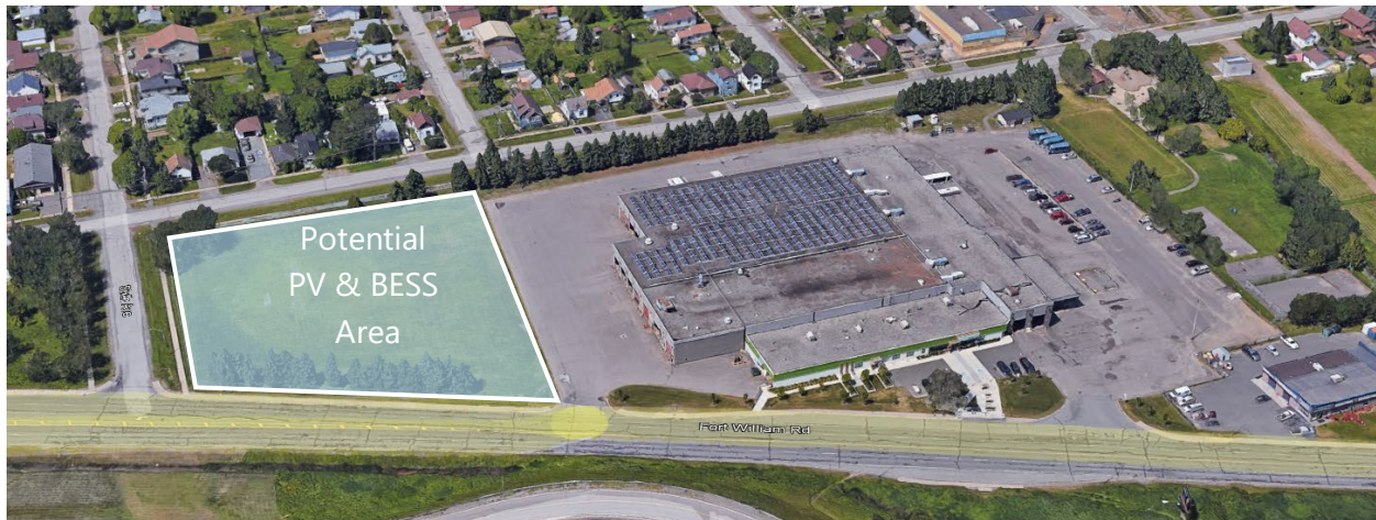
Figure 75. Aerial highlighting area where BESS could potentially be located.
