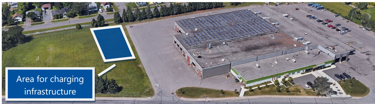
Figure 56. Fort William Transit Garage outdoor area for charging infrastructure.
