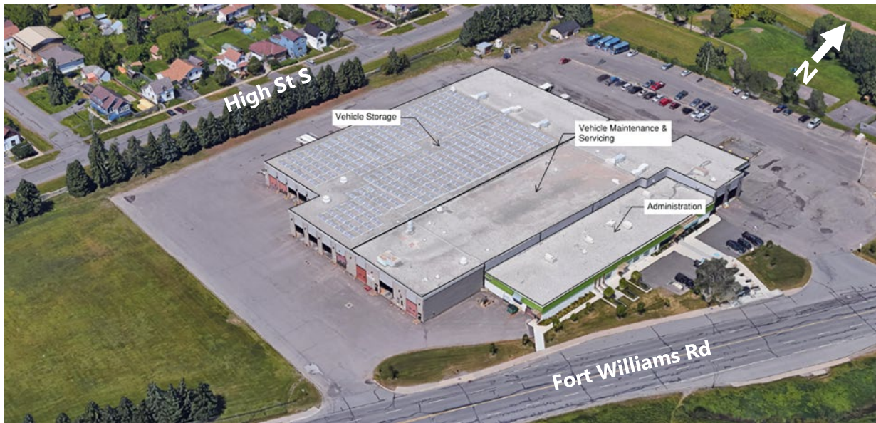
Figure 42. Fort William Road Transit Garage
