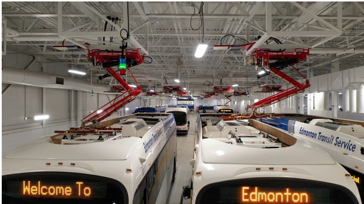
Figure 51. Example of ETS in-depot pantograph chargers
