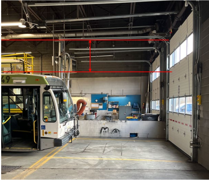
Figure 70. Overhead Clearance at Fort William Road Transit Garage
