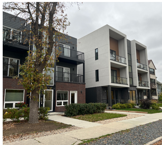
Building designs should avoid blank facades along ground floors through the use of fenestration, canopies, and other design and massing details.
