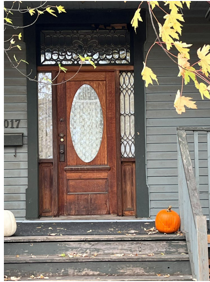
Photograph 16: Close-up of the front entrance featuring original wood front door with square-headed transom and sidelights (Source: Egis, October 15, 2025).
