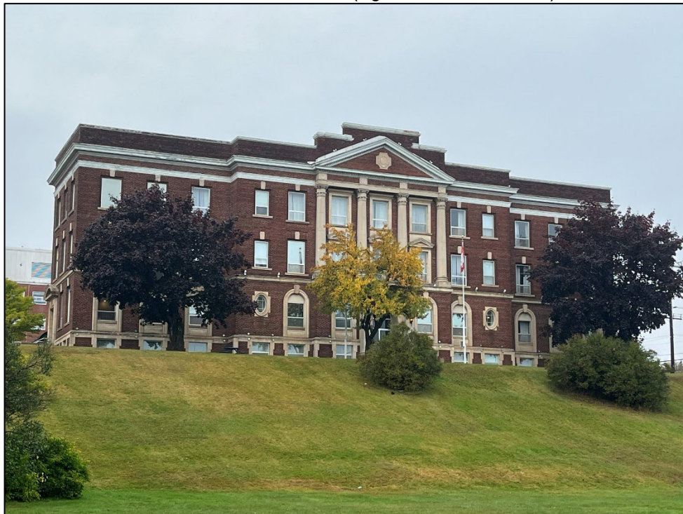
Photograph 2: East elevation of the former Courthouse (Egis, October 17, 2025).
