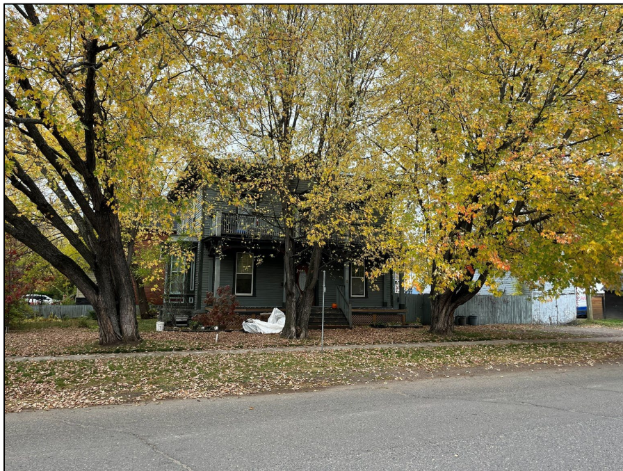
Photograph 1: South (front) elevation of 1017 Isabella Street East (Source: Egis, October 15, 2025).
