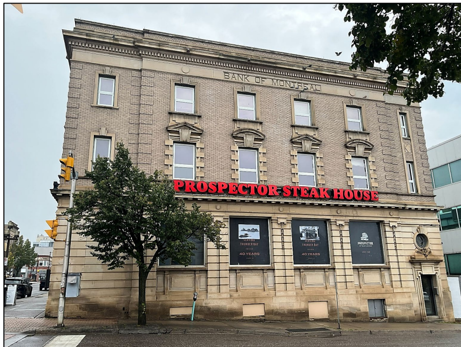
Photograph 3: South elevation (former entrance to the upper-level offices and residence) of the building (Source: Egis, October 17, 2025).
