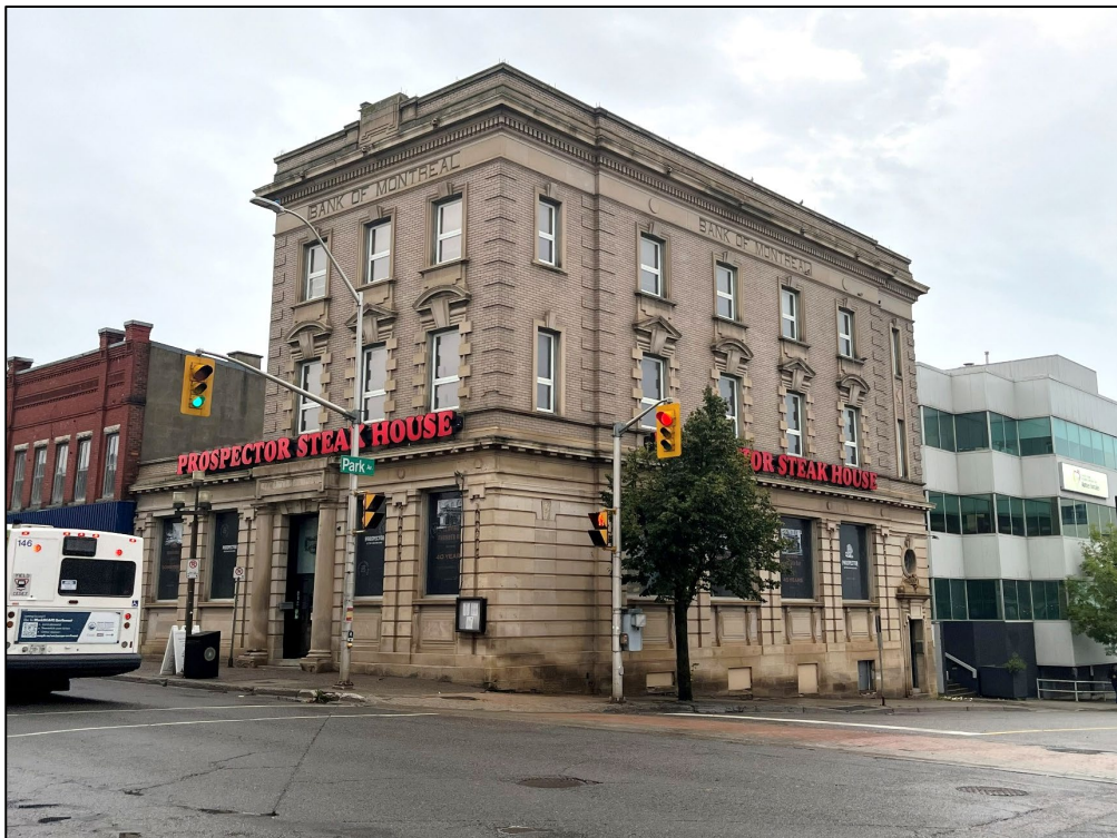
Photograph 1: West (former bank entrance) and south (former office/residential entrance) elevations of the former bank building (Source: Egis, October 17, 2025).
