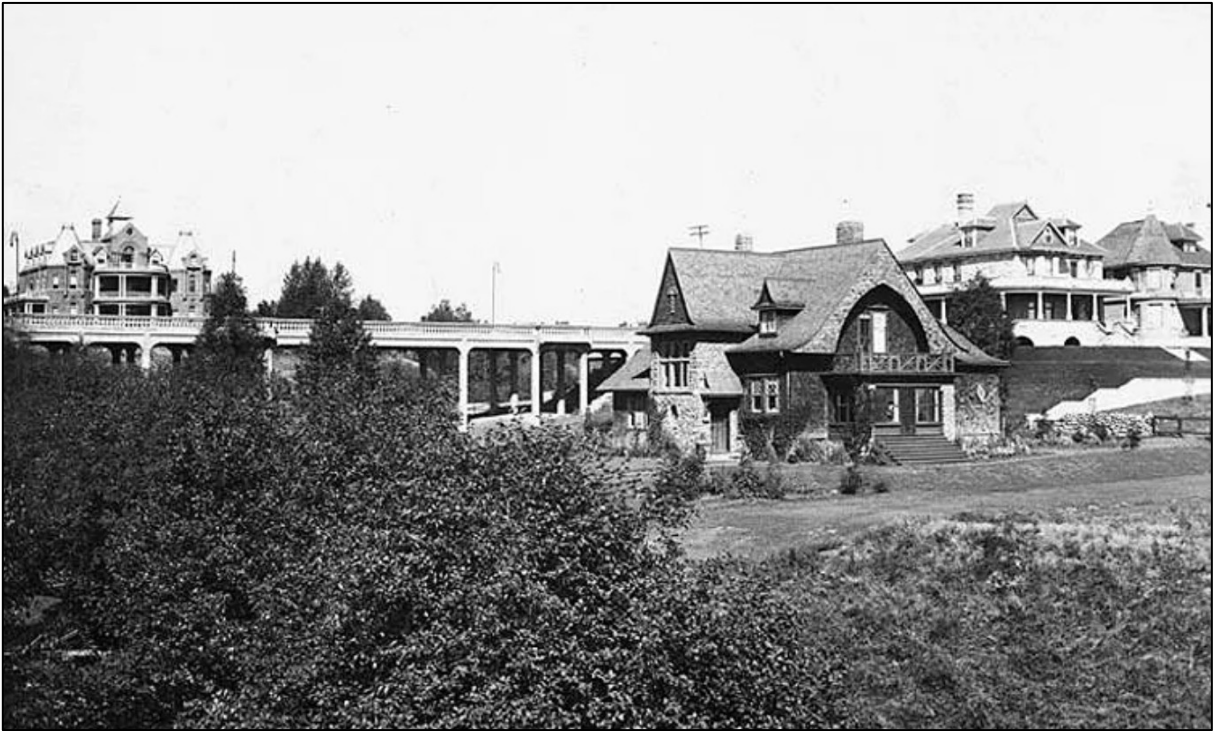
Image 1: ca. 1910 photograph of the east and south elevations of the house (Source: Thunder Bay Museum)
