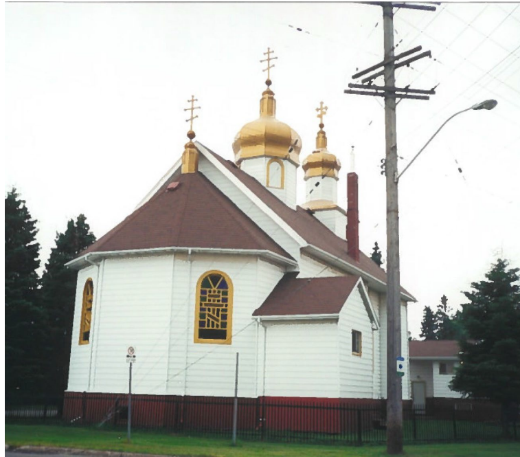
Image 4: Colour photograph of the church after renovations (Source: City of Thunder Bay)
