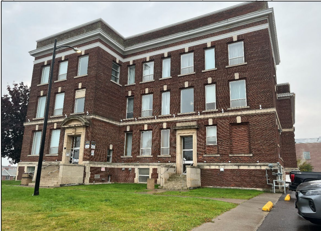
Photograph 4: View of the north elevation showing side entrances including lobby entrance on the south side (Egis, October 17, 2025).
