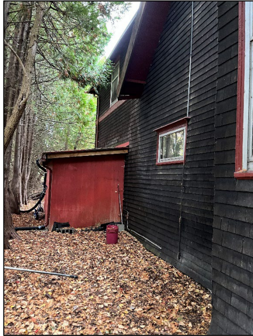
Photograph 8: West elevation, looking north (Egis, October 16, 2025).
