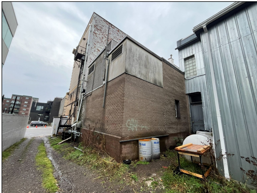
Photograph 5: East and north elevations of the rear of the building (Source: Egis, October 17, 2025).
