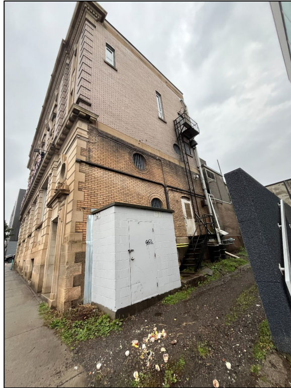
Photograph 4: East elevation (rear) of the building (Source: Egis, October 17, 2025).
