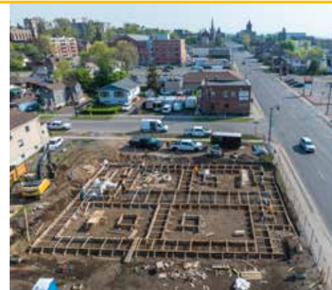
Photo of the construction of an 18-unit apartment building being constructed along Algoma Street. This project was a successful recipient of funding through the Housing Accelerator Fund program.
